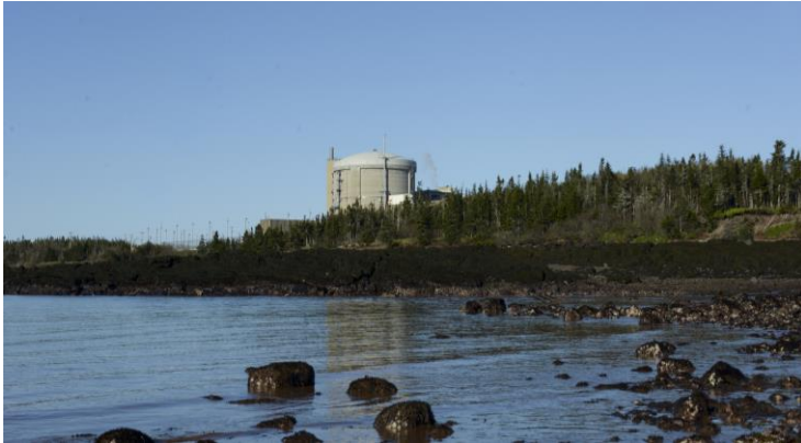
Point Lepreau – 700MW nuclear
